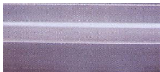
Steel girder - after
